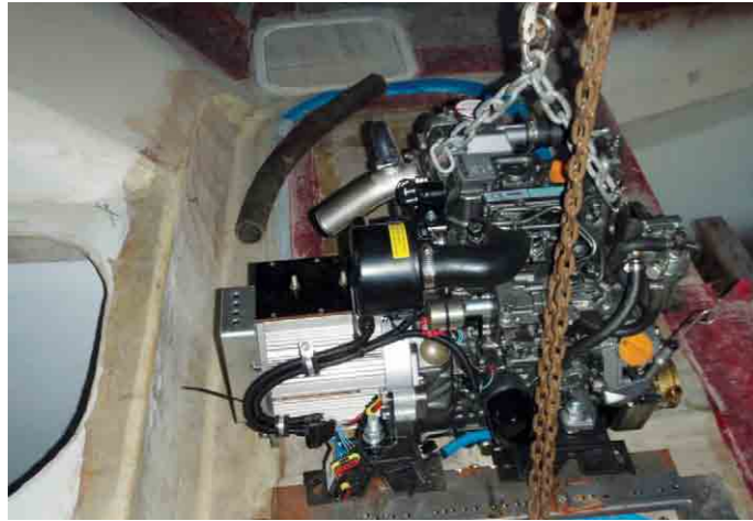
Diesel generator being lowered into position. (above left)
